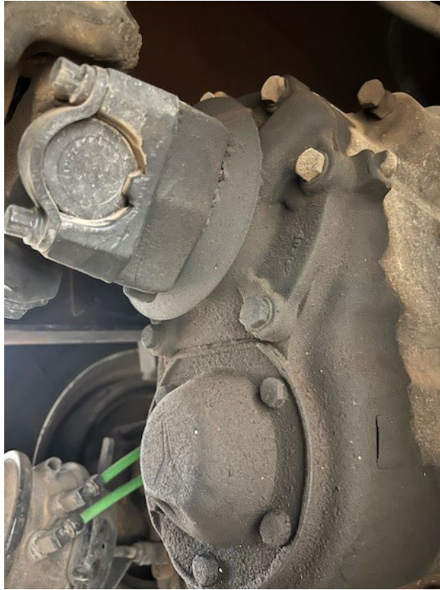
Pinion Seal Leak
