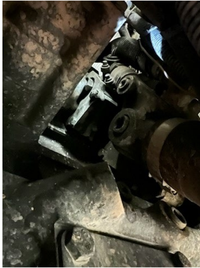
Coolant Leak at Oil Cooler
