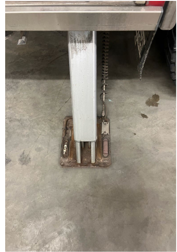
Missing and non Working Safety Lights for Outriggers
